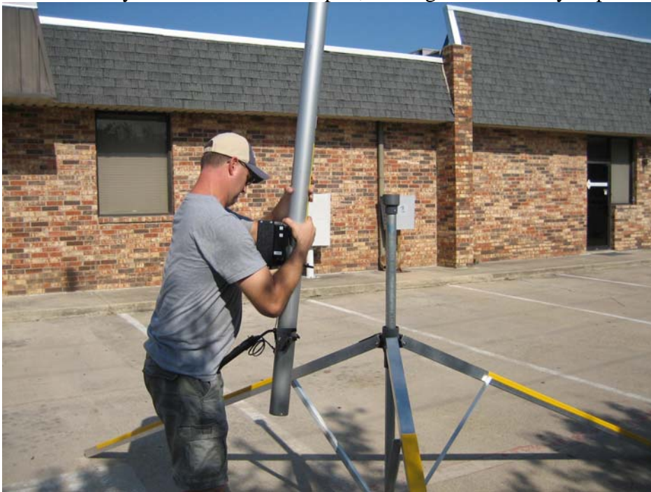
Picture of the mast section being placed on the tripod.
