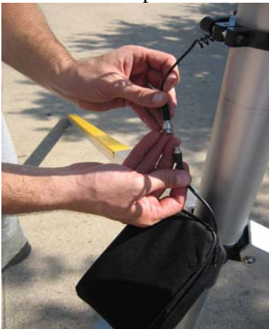
Picture of connection from Battery to Monitor assembly box.
