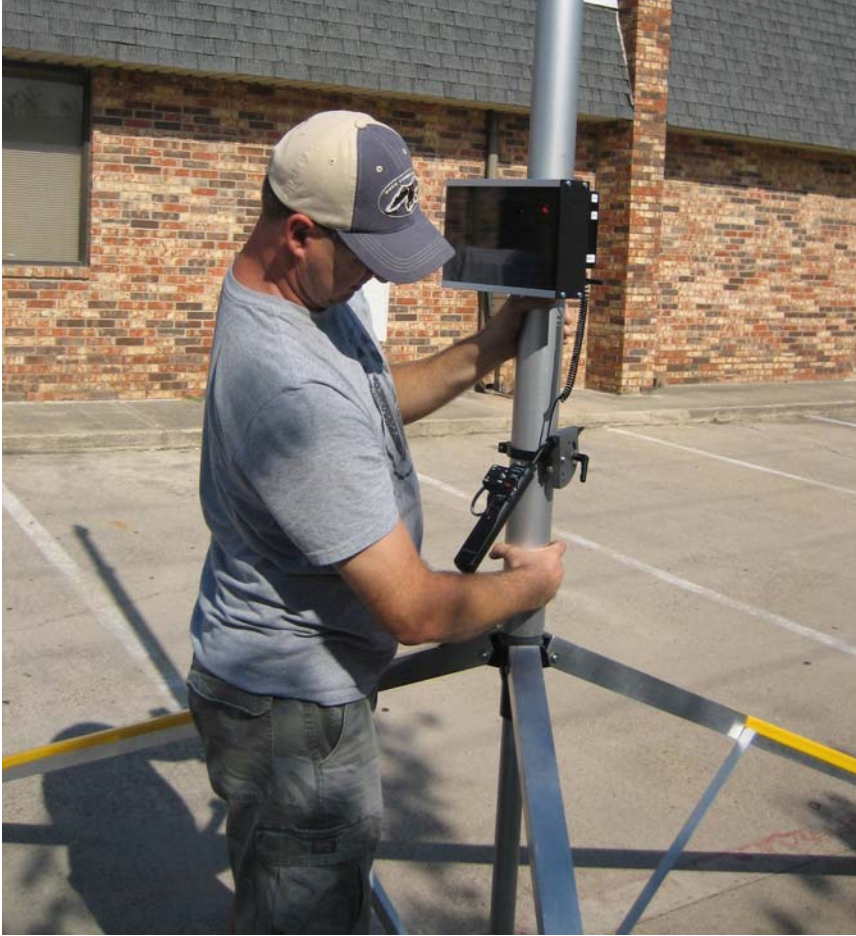
Picture of Mast section in place on the tripod.
